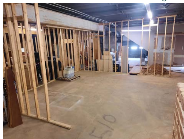
Existing framing in basement
