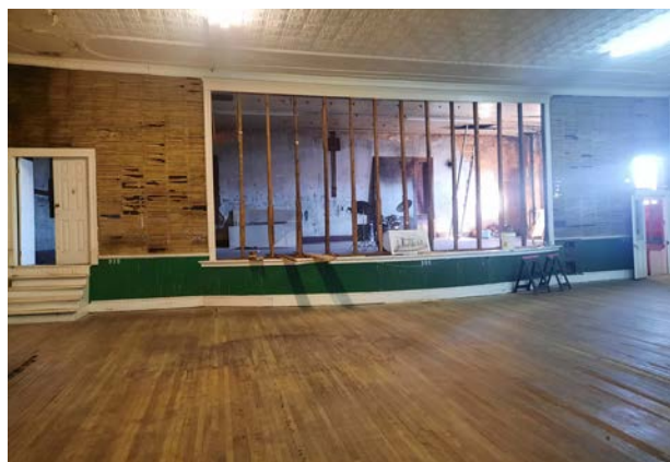
Top floor performance hall stage
